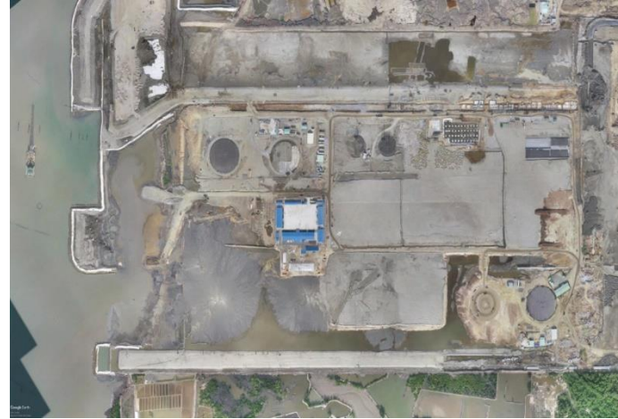
Tank farm area
