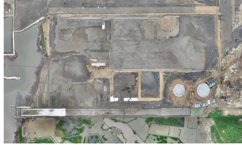
Overall Tank Farm Area
