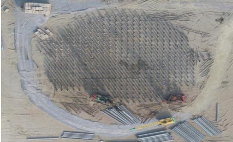
Piling Work at LPG Tank
