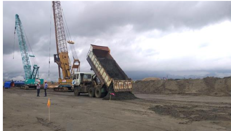
Olefin plant construction
